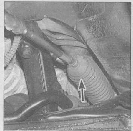
24.9b Check each steering gear boot (arrow) for cracks and leaking steering fluid
